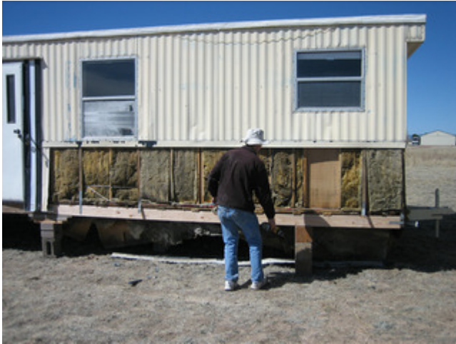
Ops trailer damage repaired.
